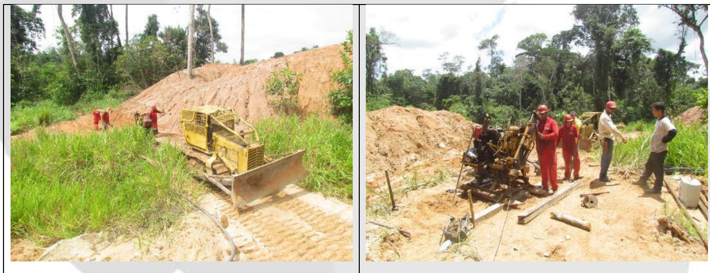
Figure 3 - Drill Pad Preparation at the Daniel target
