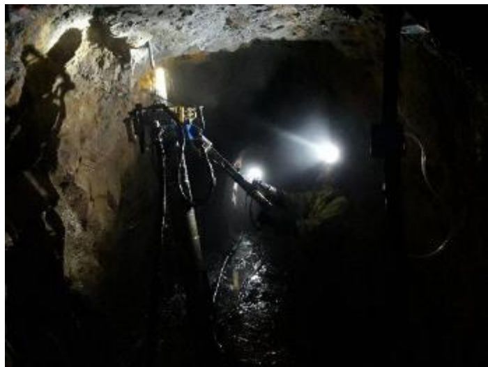
Figure 4 - installation of rock bolts in Keillors Crosscut
