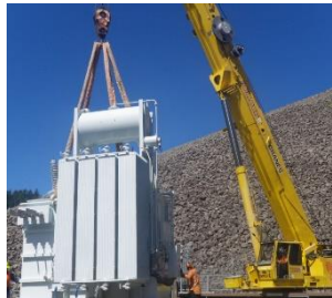
Transformer lifted onto trailer for short journey to switchyard
