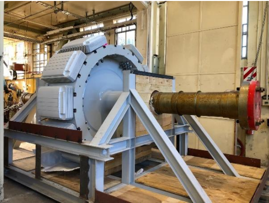
New G3 rotor awaiting installation
