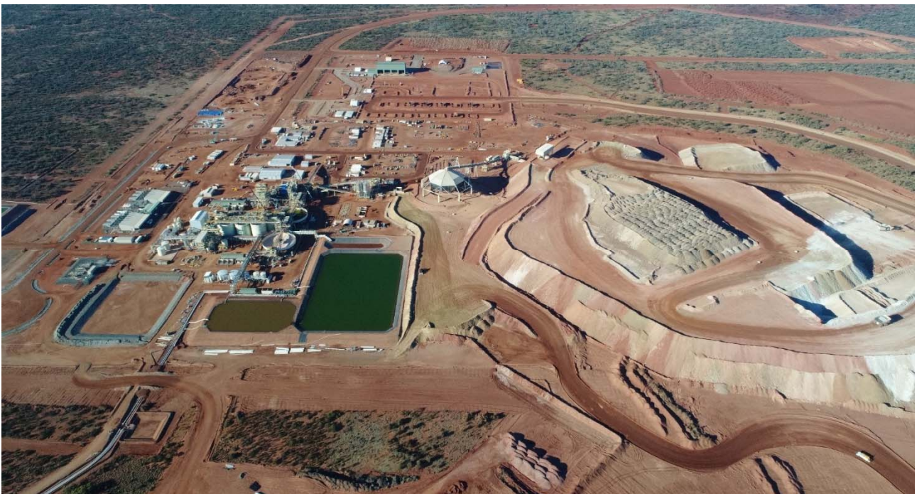
Aerial view of Gruyere process plant and infrastructure - June 2019
