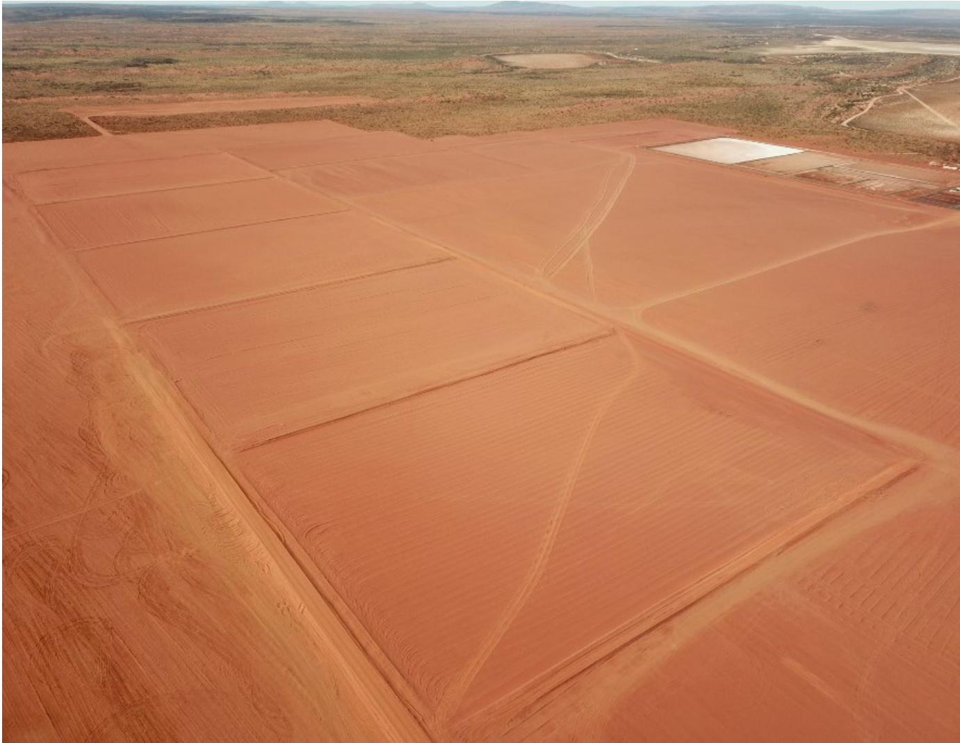
Initial Pond Earthworks Complete Ready for Liner
