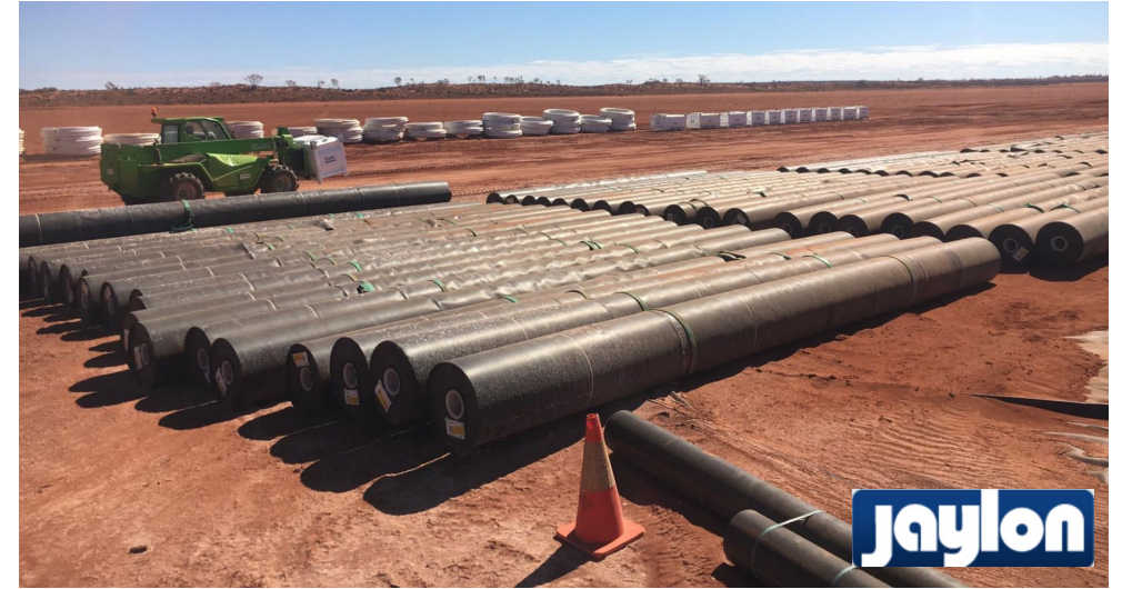
Liner Delivered to Site
