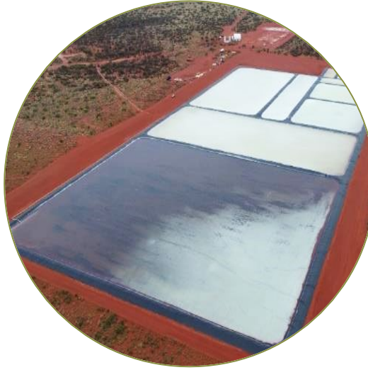
Brine Solar Evaporation Located in high evaporation region ~3,800mm
