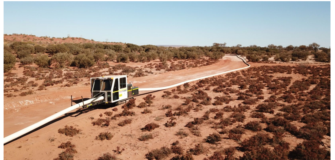
Pipeline Installation Progressing
