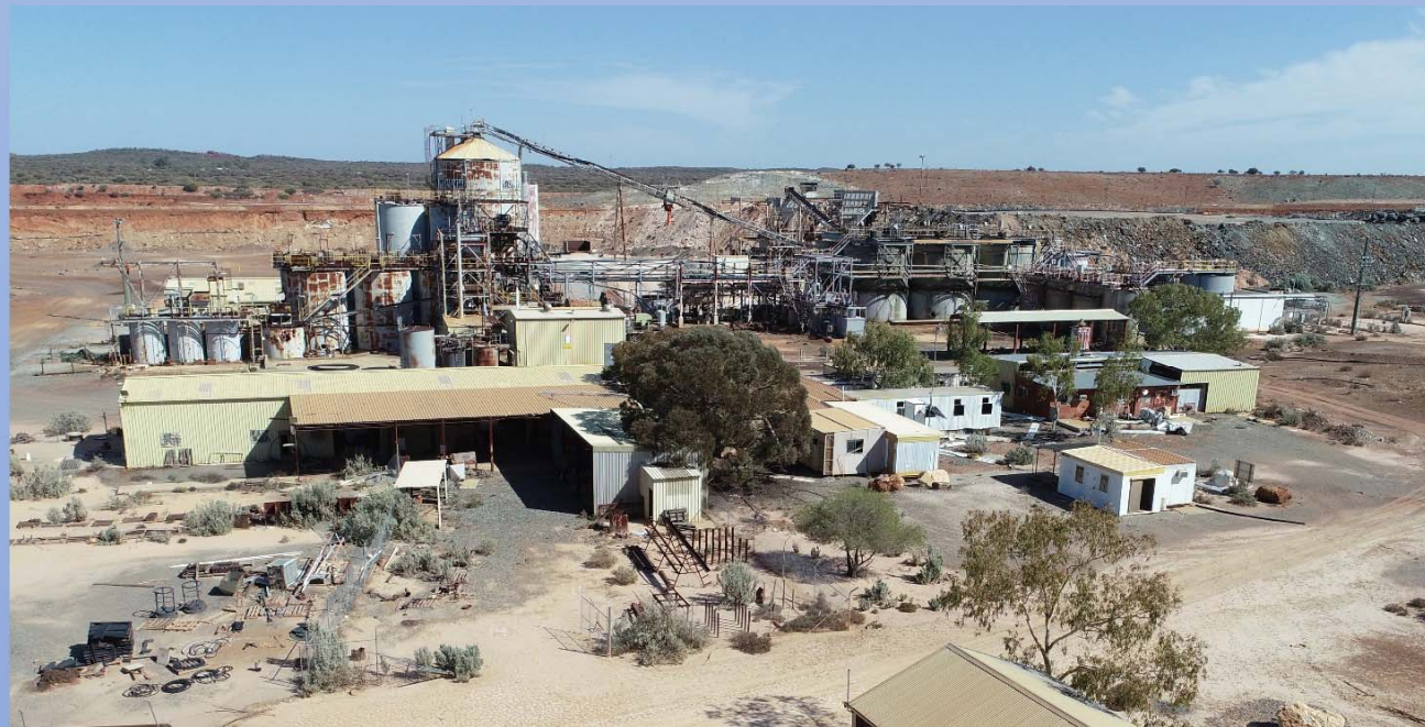
Youanmi Gold Mine Infrastructure
