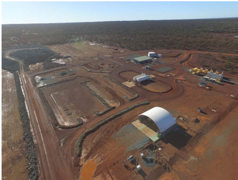
Figure 2: Monty Project surface facilities.
