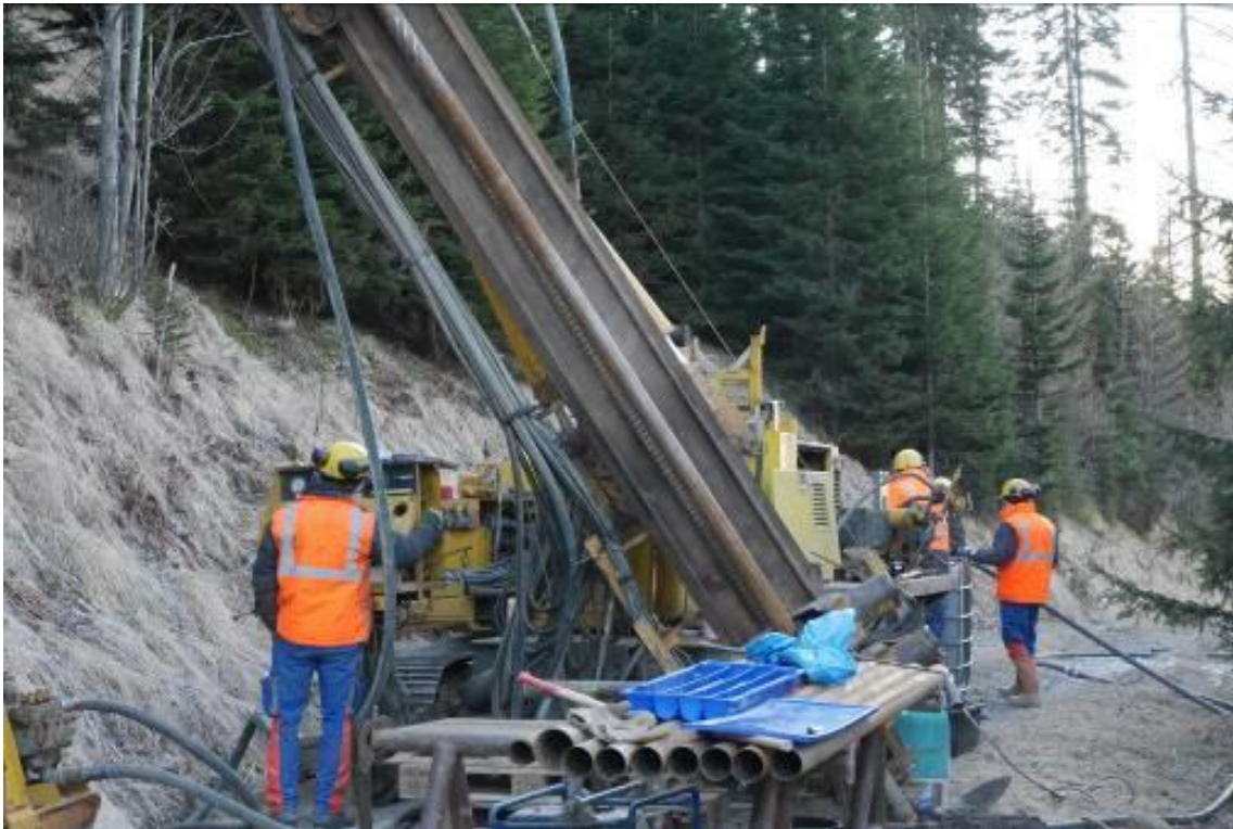
Figure 1: Atlas Copco (Mustang A66CBT) at Drilling Borehole Number P15-1.
