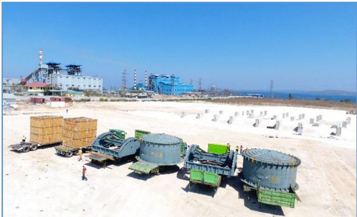
Figure 1: The furnaces arrive showing the power station in the background.
