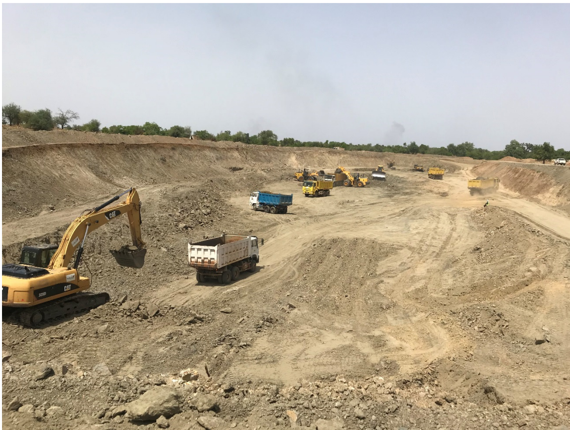
Photo 1: Water Storage Pit at M5
