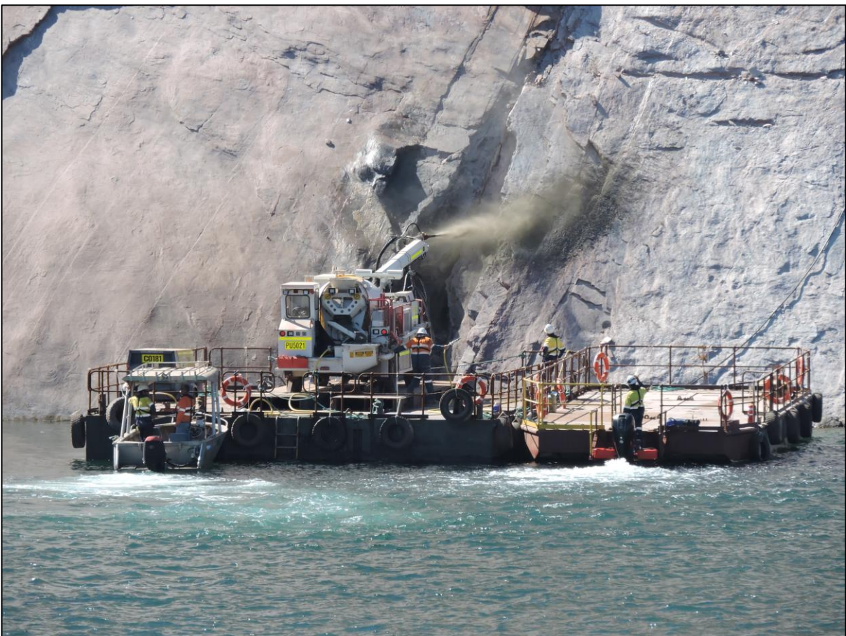
Figure 7: Shotcreting of Main Pit Footwall – July 2018
