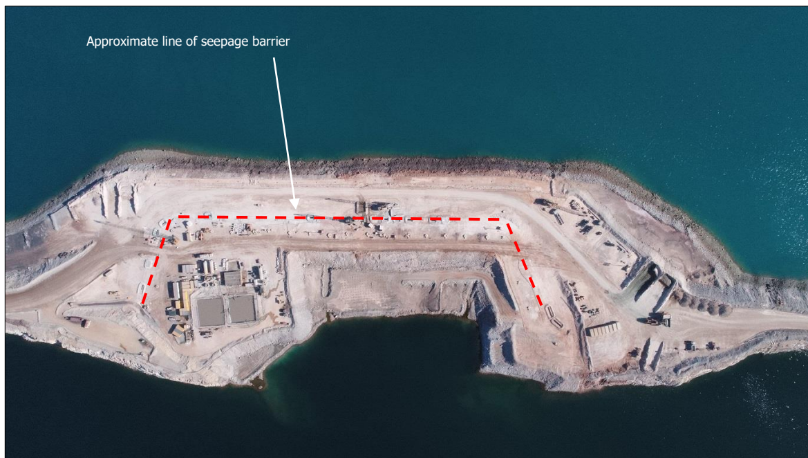
Figure 2: Aerial view of seawall embankment – end June 2018
