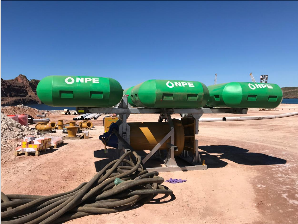
Figure 4: Submersible dewatering pump ready for commissioning - July 2018
