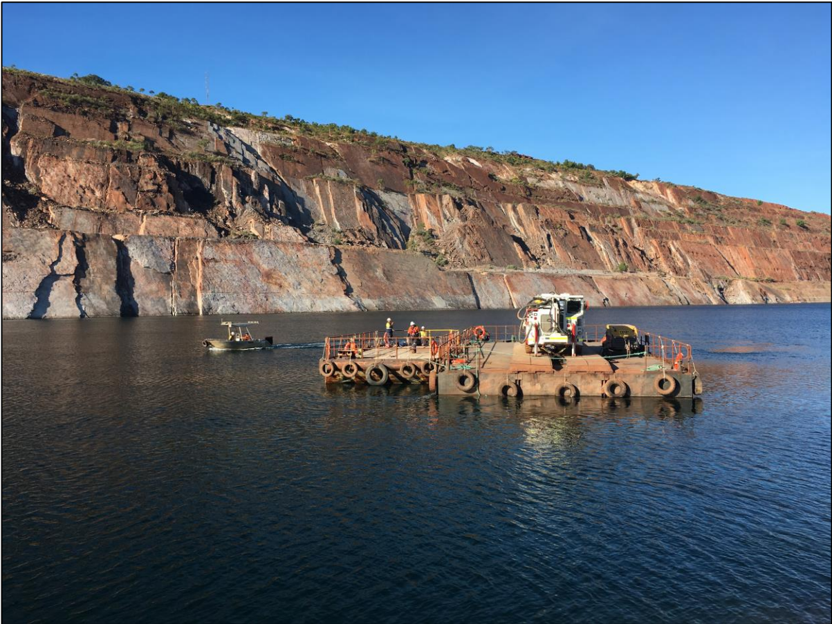
Figure 6: Deployment of barge-mounted shotcreting equipment in Main Pit - July 2018
