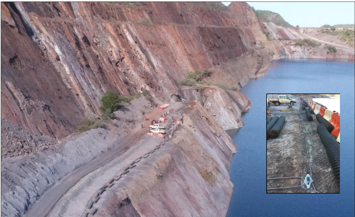
Figure 5: Avalanche mesh for installation on footwall - July 2018
