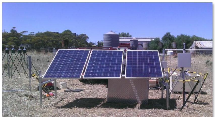
An air quality monitoring station located within the CEIP Mining Lease
