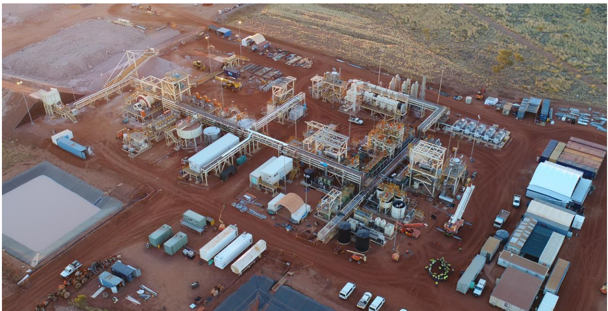
Process plant overview – 17 July 2018
