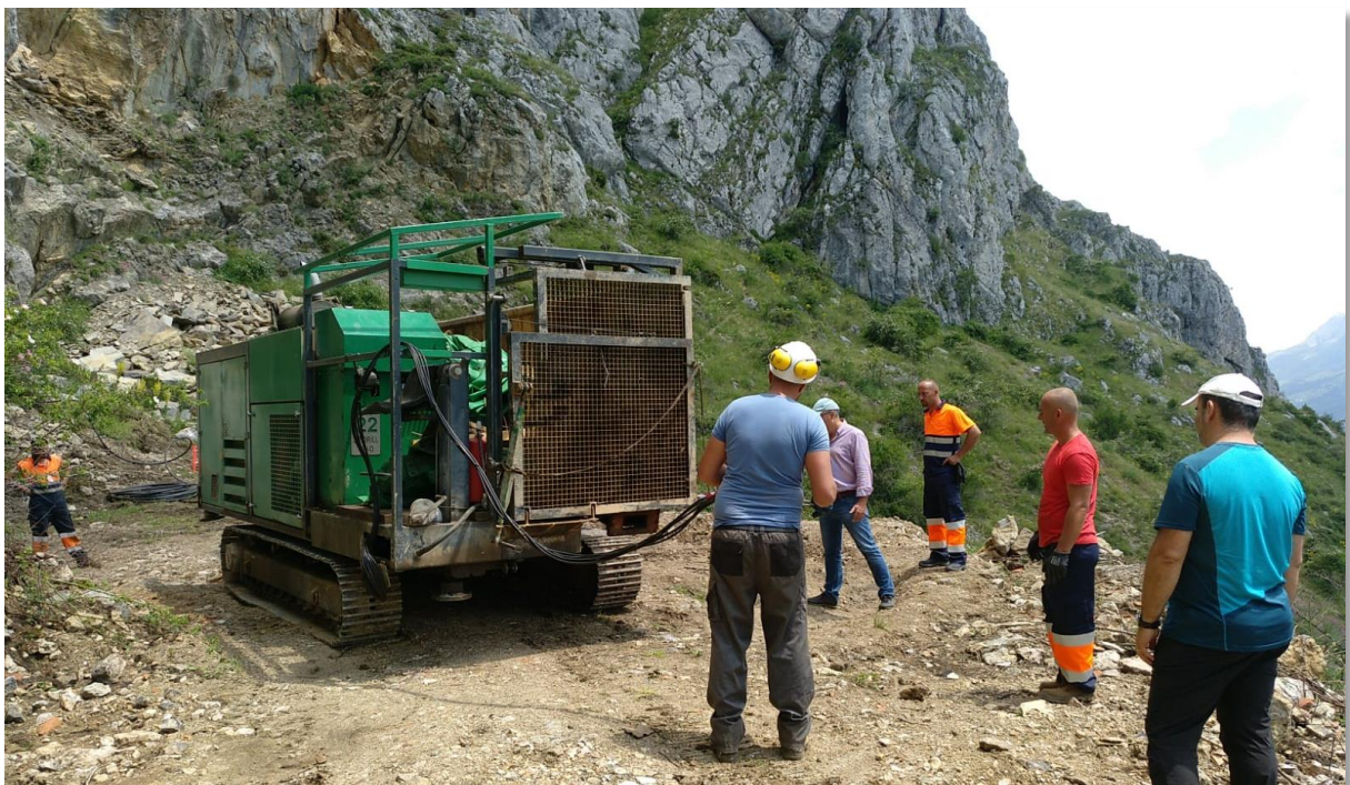
FIGURE 2. Locating drilling rig for first drill hole - Cármenes Project – Spain
