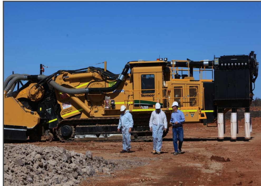
Vermeer surface miner in operation at the Centipede deposit trial mine
