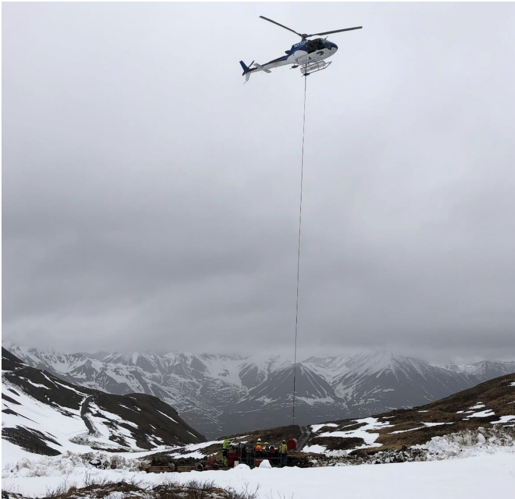
Figure 2 Helicopter slinging in fly rig components, Zackly
