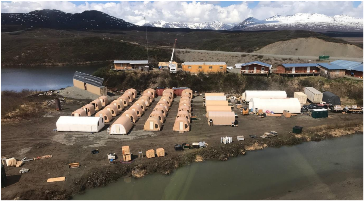
Figure 4 Exploration and drilling camp for the Alaska Range Project at nearby Maclaren River Lodge. The Zackly project is situated behind the hills in the top right of this photograph
