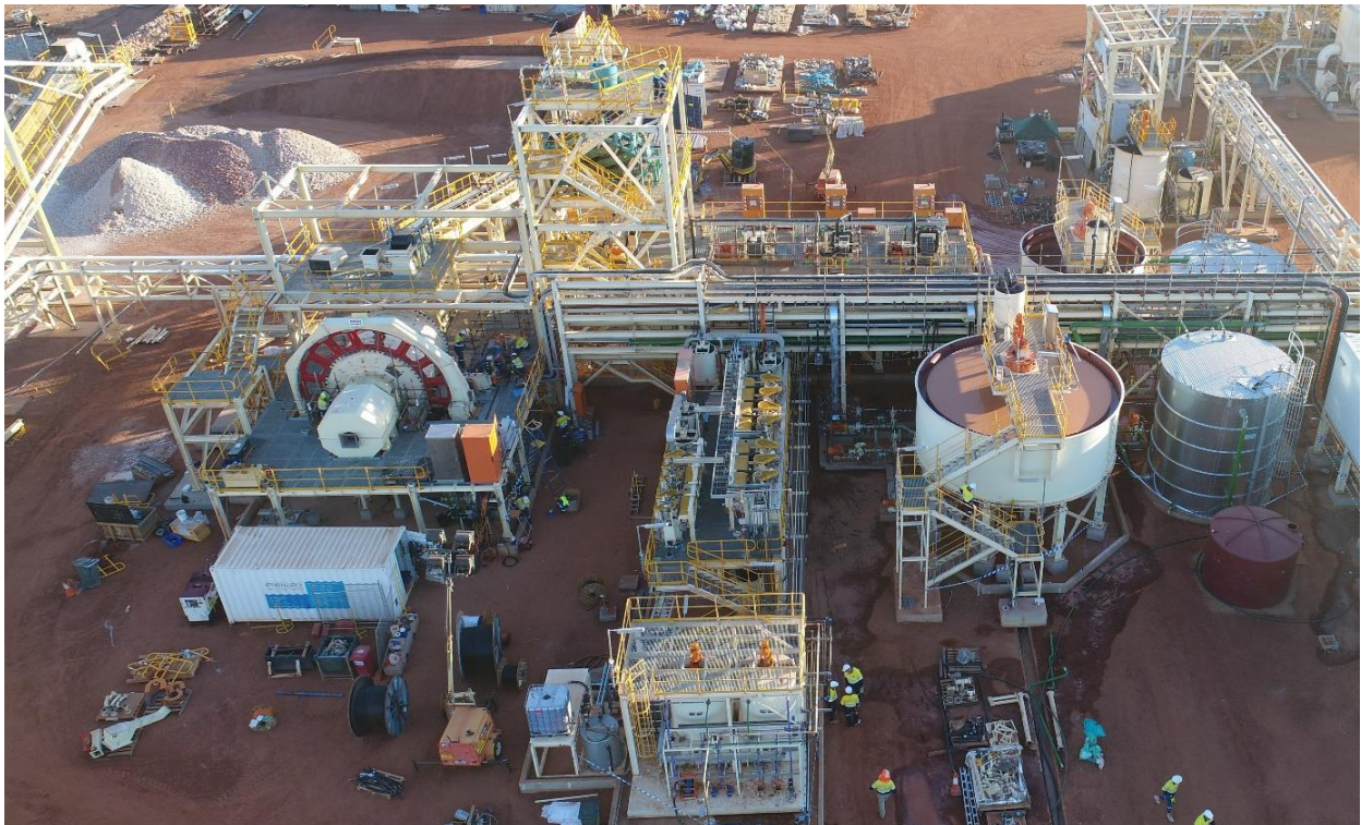
Commissioning of magnetic separation, flotation, tailings and water services
