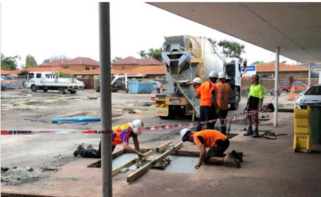
Recent site works at City Subaru
