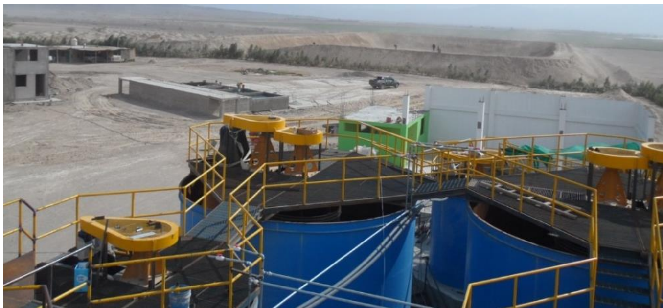
Figure 5 Vista carbon and leaching tanks, with tailings dam in the distance
