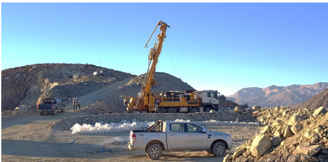
RC drilling activities advancing well at the San Antonio copper mine in Chile
