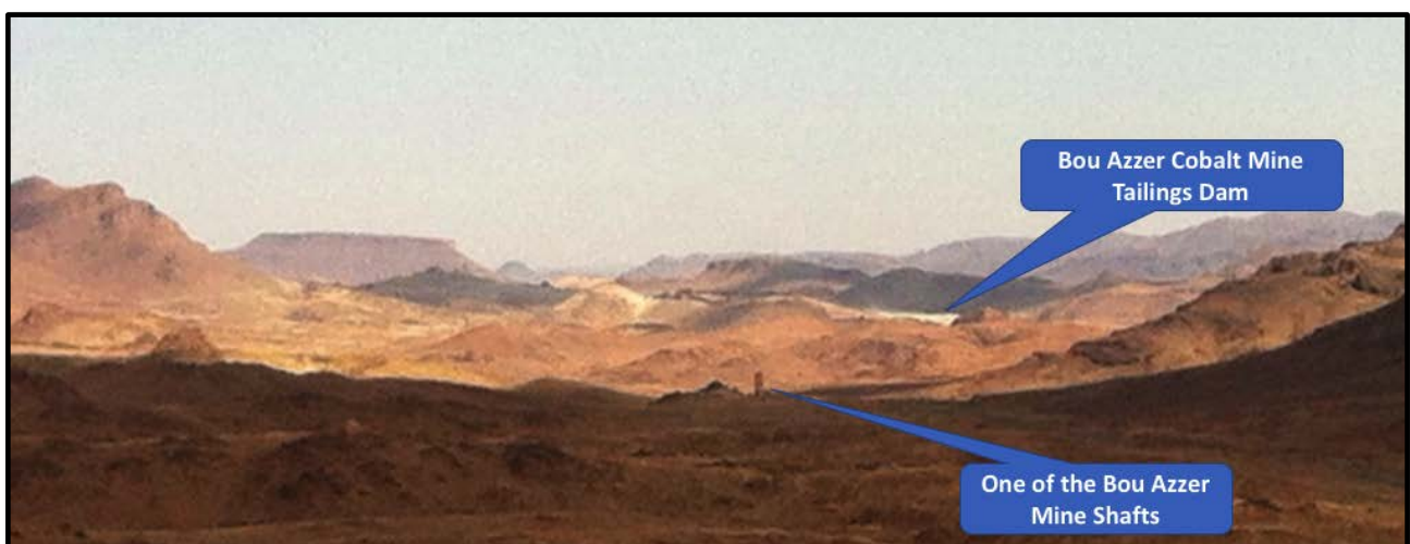
Figure 1: The Bou Azzer Cobalt Mine taken from the Bou Amzil Licence looking east.
