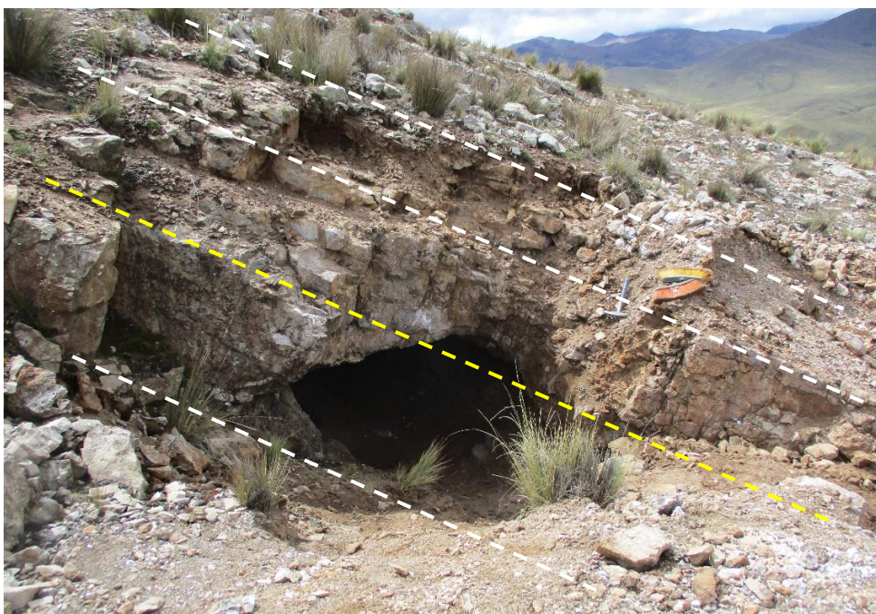
Figure 1 LEFT : Entrance to Mine 4548. The plain of the manto is indicated by a dotted yellow line. Note that the manto is concordant (parallel) to the bedding of the limestone (dotted white lines). This is characteristic of manto mineralisation.
