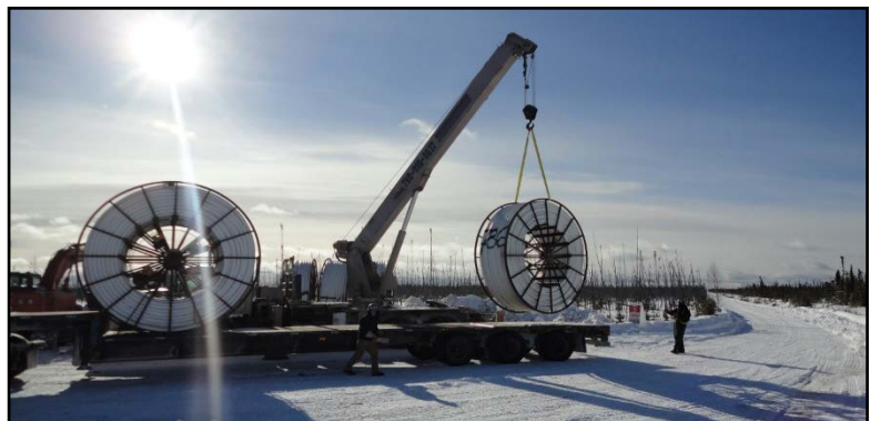
Figure 3 – PLJV Thornbury Reactivation Project Pipeline Installation
