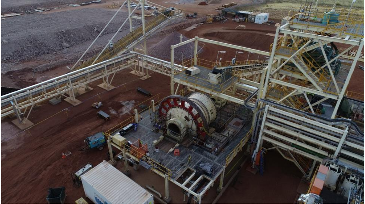
Mill girth gear installed
