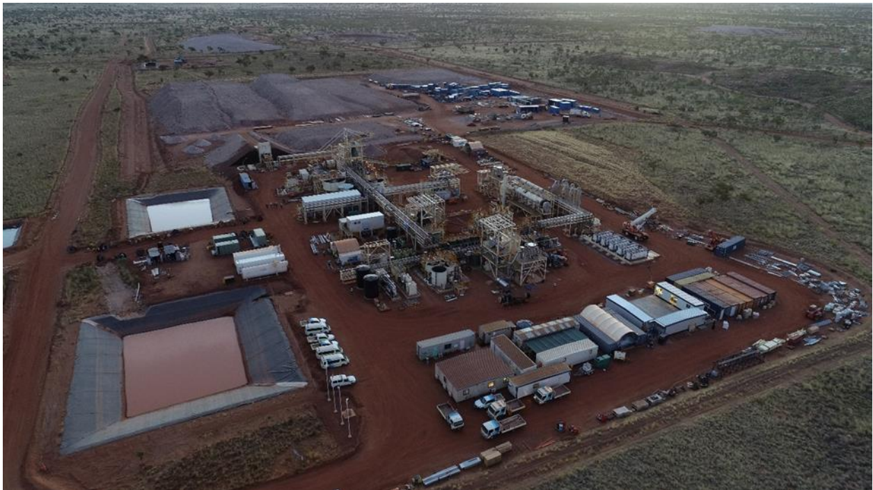
Process plant overview – 21 May
