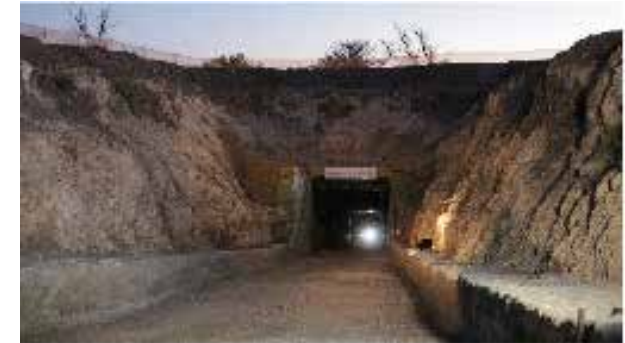
Surface portal access
