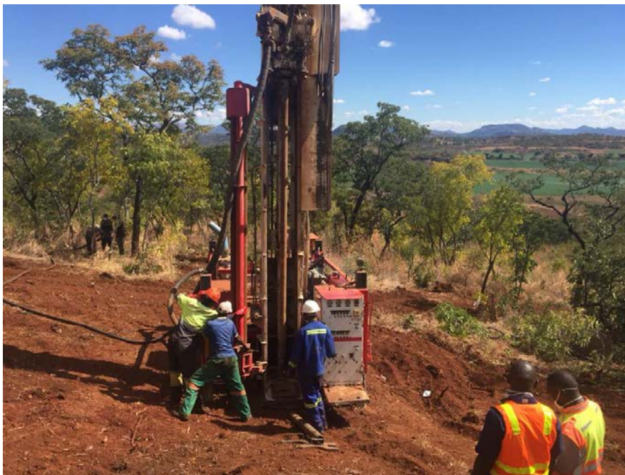
Figure 1: Drilling rig at cleared drill pad in Bonnyvale
