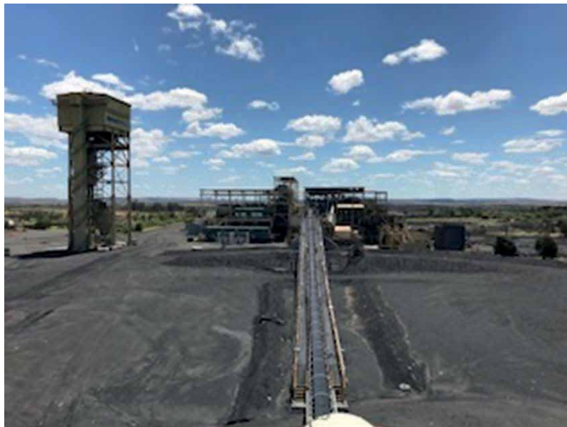
Figure 7-3 : View of Coal Preparation Plant from Stockpile Feed Hopper
