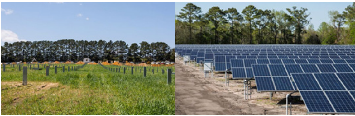
Church Road and Hanover under construction
