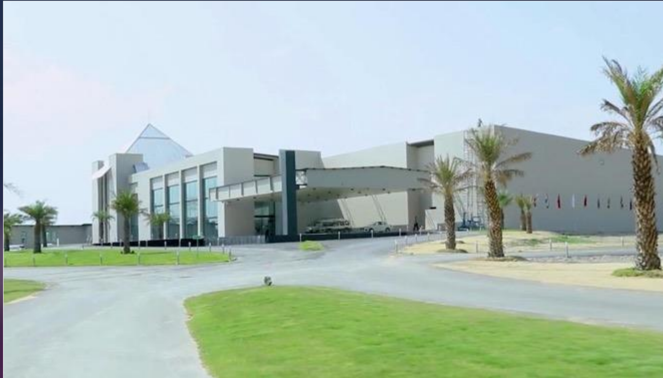
Approach to the Main Building - Hotel & Casino & Retail
